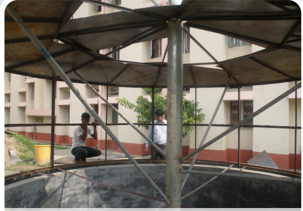
Installation of Biomethanation Plant_ A learning
