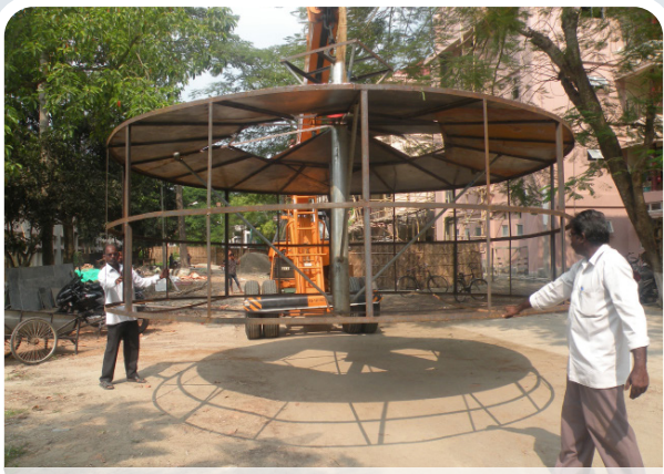
Installation of Biomethanation Plant_ A learning
